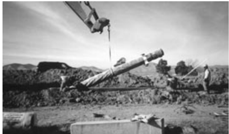
Zone 1 Water Line Replacement Project Construction
